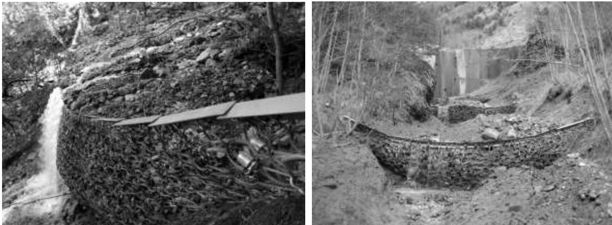
**Fig. 2** Filled barrier in Porainé Spain 2010 (left) and 3 filled barriers as erosion control in Merdenson, Switzerland.
